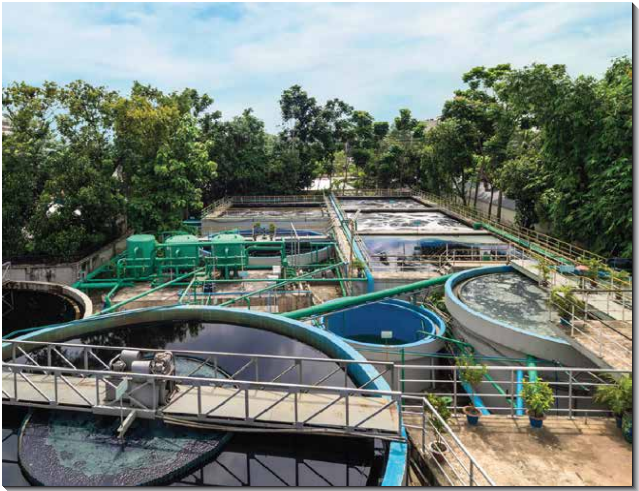
ETP Plant for Safe Environment
