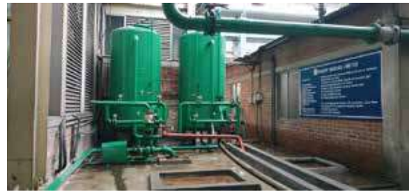
Image of Utility water recycle technology to use treated water for process.
